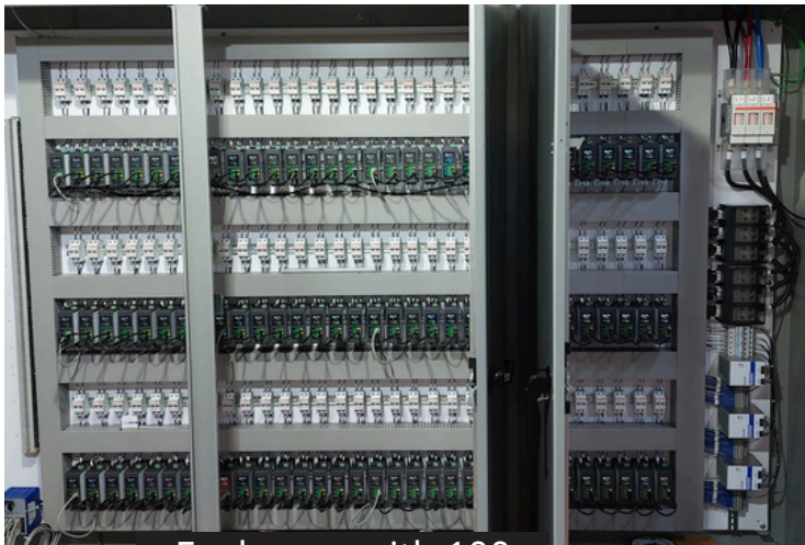
Enclosure with 100 Eurotherm EPacks
